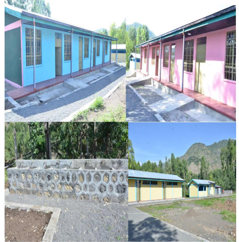
Robit Inclusive Schools Construction
